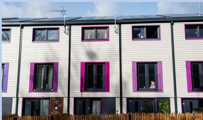
Figure 16. Insulated façade installed in Nottingham 2017, the first Energiesprong demonstrator in the UK.
