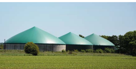
Figure 27. Gas storage associated with anaerobic digestion plant. Image courtesy of Spielvogel.
